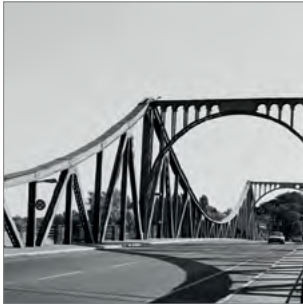
S-P01 Glinicker Brücke
